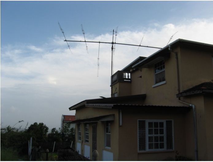
FROM CARL 8P6OP IN BARBADOS. ANTENNA HAS DAMAGE FROM HURRICANE TOMAS.
